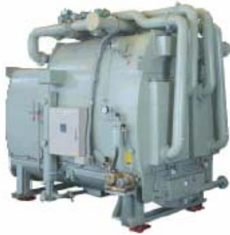
Figure 11: Nishiyodo adsorption chiller (HIJC Inc, 2007).
